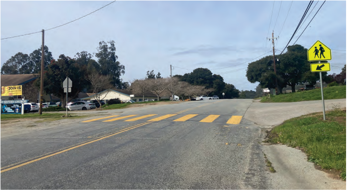
Crosswalk leading to Prunedale Elementary School.
