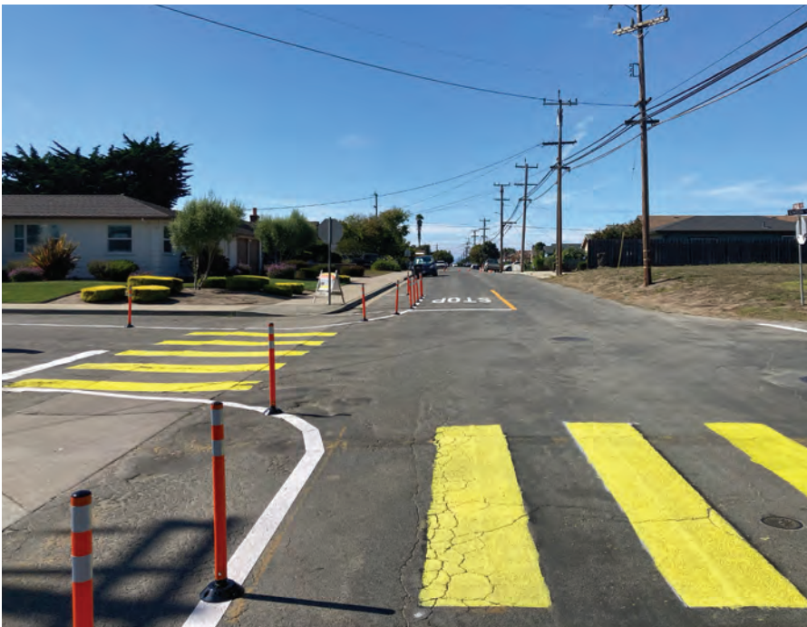
Figure 5. High visibility crosswalks and curb extensions at Geil & Union
