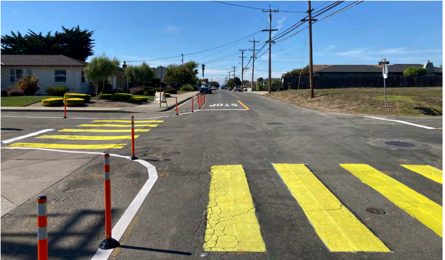
Temporary installation at Union Street & Geil Street.
