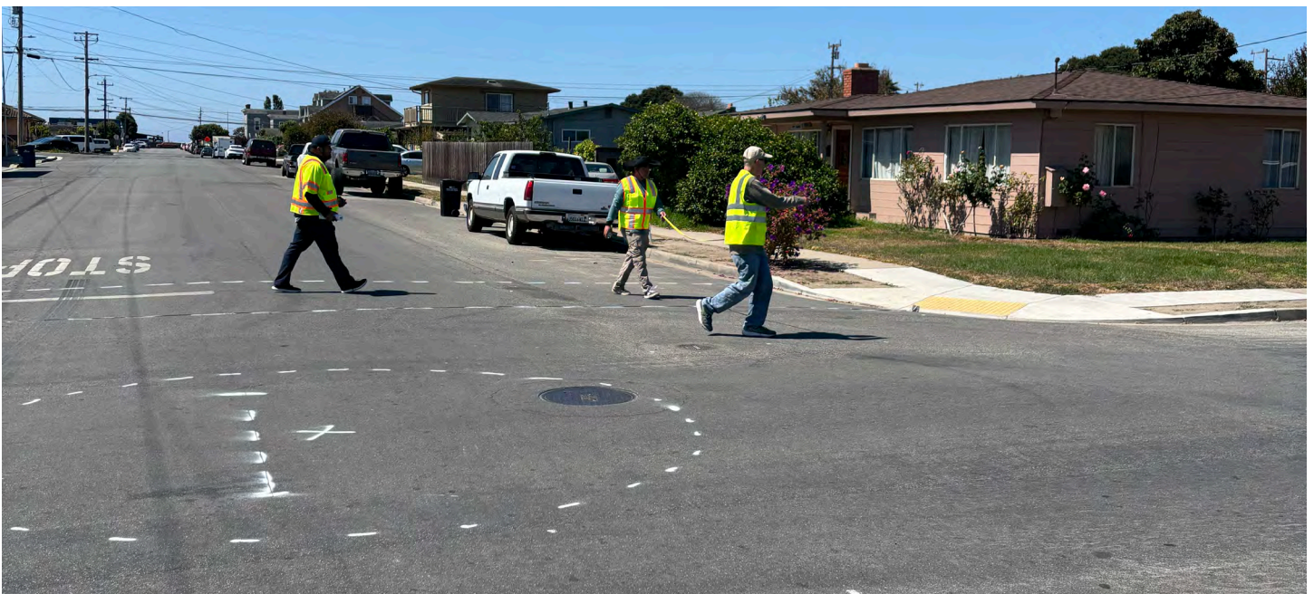
Project team working on the temporary installations in Castroville.
