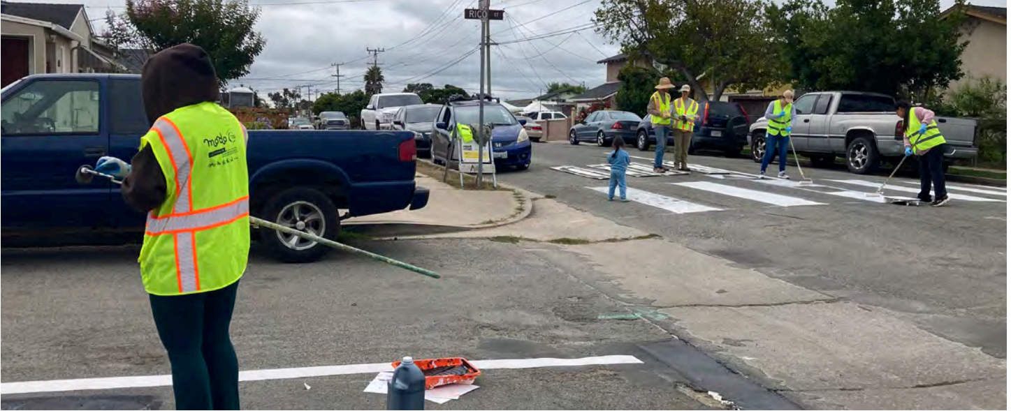
Project team installing a crosswalk.
