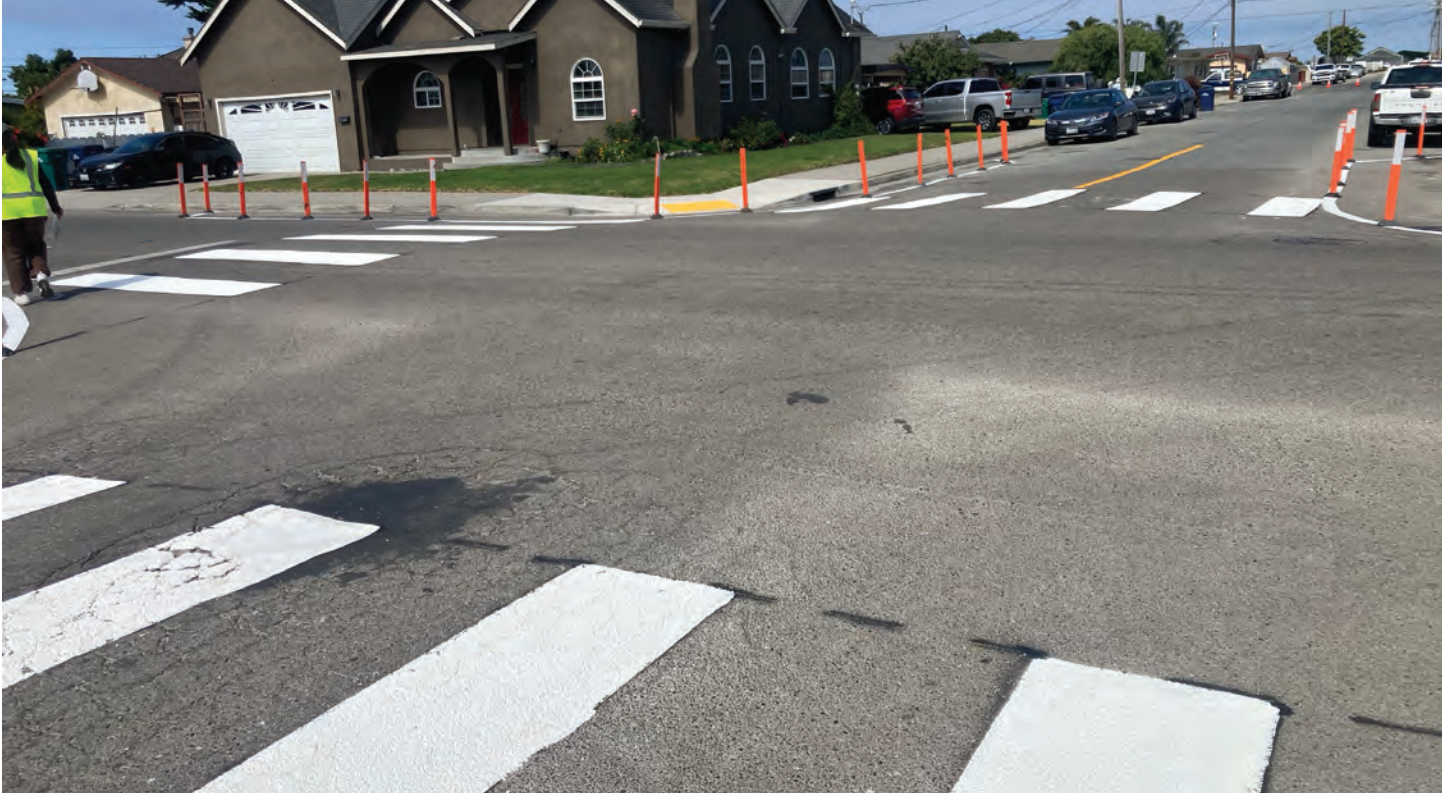
Figure 3. Temporary high visibility crosswalks and curb extension on Geil & Cooper
