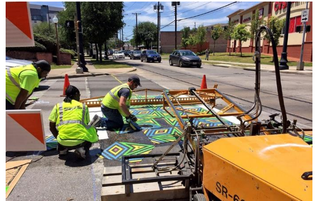
Figure 6: Thermoplastic Installation
